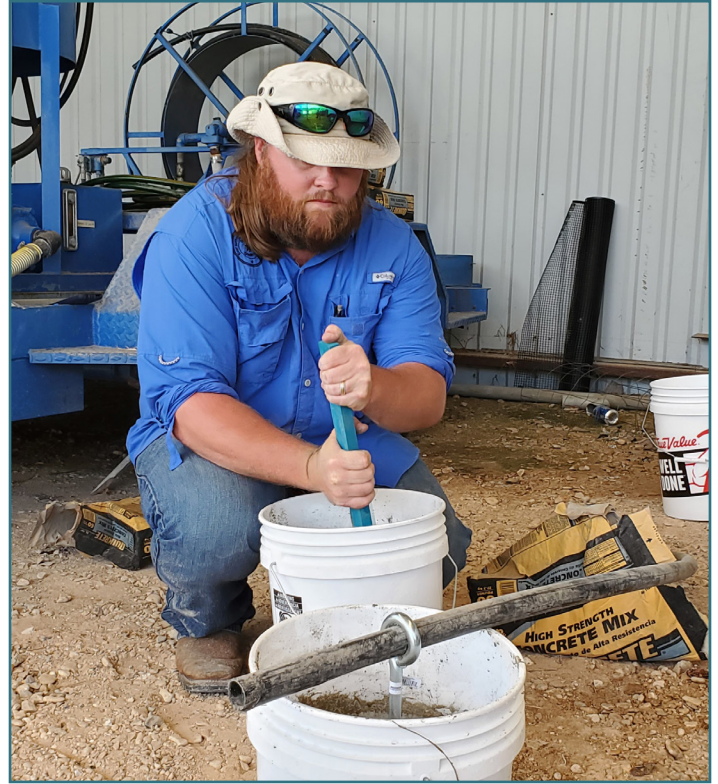
Constructing anchors for No Wake Buoys for Medina Lake.
