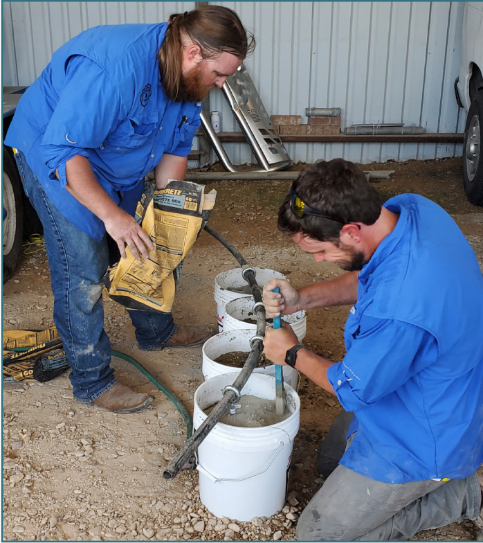
Constructing anchors for No Wake Buoys for Medina Lake.
