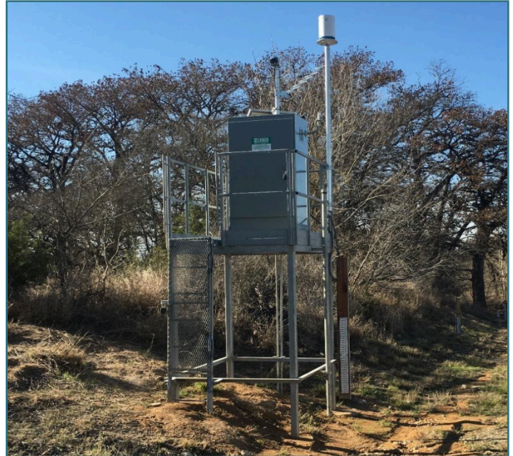
USGS Stream Gage at Sabinal River Bridge at Utopia, TX FM-1050, 08197970 Sabinal Rv at Utopia, TX. Photo taken March 4, 2020. Stream Gage is located on the Left Bank-Downstream side of the bridge near the top of the stream bank.
